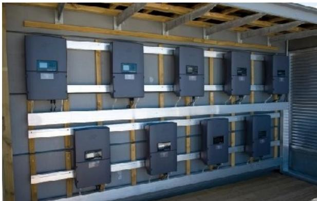
**Figure 2:** Here we see a bank of string inverters on a garage wall. As is clear, string inverters are big and heavy and not something you would put on your roof.
